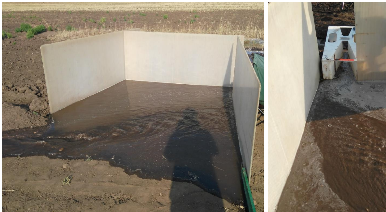
Obr. 11: Instalace Parshallova žlabu
